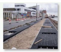
Minimize subgrade compaction by dissipating heavy urban loads throughout the structural ArborRaft.
