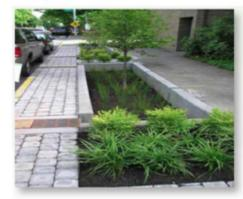
Maximizes shallow storage and conveyance assuring the best bio-swale efficiency.
